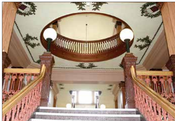
In the center of the courthouse's second-floor rotunda is a 14-foot diameter hole encircled by an ornamental balustrade.
